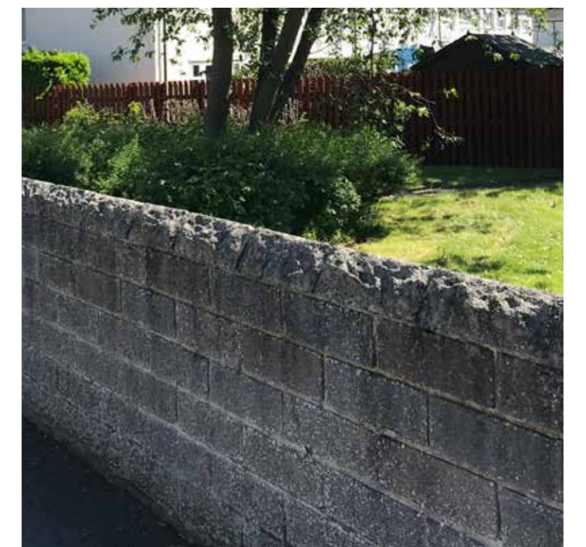
boundary wall repairs
