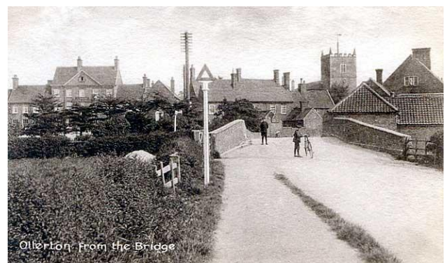
Fig.8 Ollerton from the bridge c.1920
