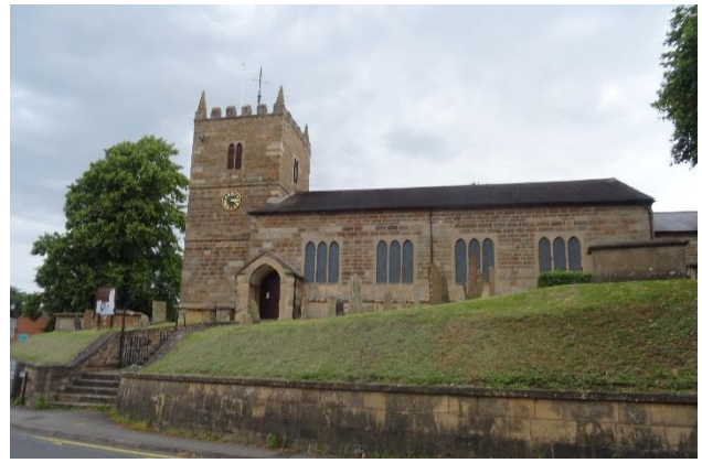
Fig.15 Church of St Giles – stonework and ashlar
