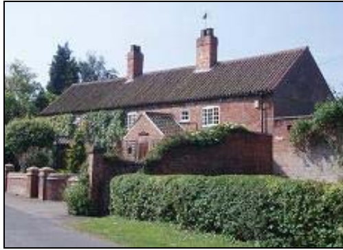
Apple Tree Cottage and Fleet Cottage on Holme Lane characterise this character zone with their simple plan form, traditional materials and traditional fenestration
