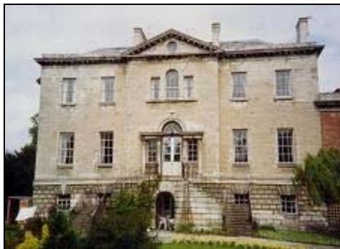
Winthorpe Hall, the principal house in the village, built in the Classical style using a projecting central pediment and Venetian windows and doors to the second and first floor. The use of the rusticated masonry on the ground floor and steps up to the first floor distinguishes the first floor as the principal floor, known as the piano nobile .
