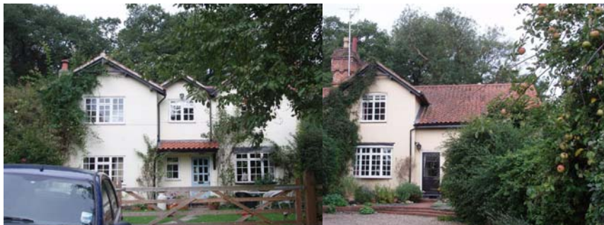
8 – 9 The Drive today, showing how much the buildings have been altered. Successive extensions have caused the original form of the buildings to lose its symmetry (most notable in the two new gables on the left), the exposed brickwork and stone dressings have been painted over and the window shape and glazing pattern have also been lost.
