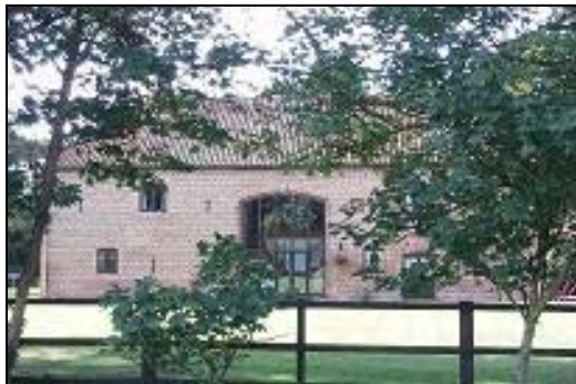
Converted former threshing barn on Hargon Lane, one of the few surviving former agricultural buildings within Winthorpe
