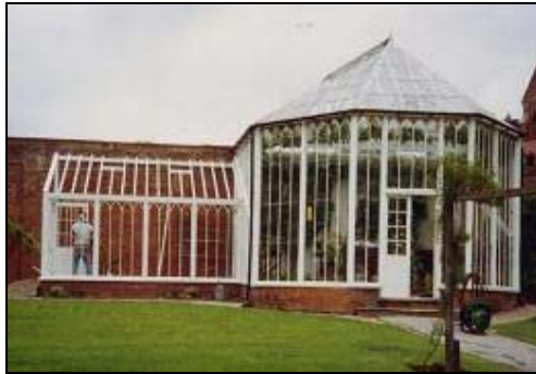
Gothick style glass houses at The Grove use a pointed arched frame with yellow glass at the apex.
