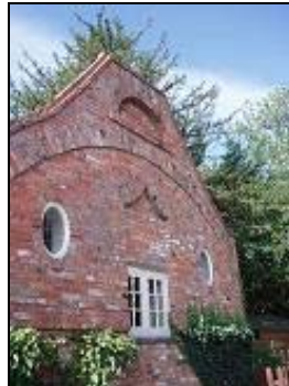
The Dairy on Gainsborough Road, associated with The Hall, is a simple vernacular building, but distinguished by interesting decorative detail on the gable end
