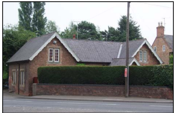
The Former School
