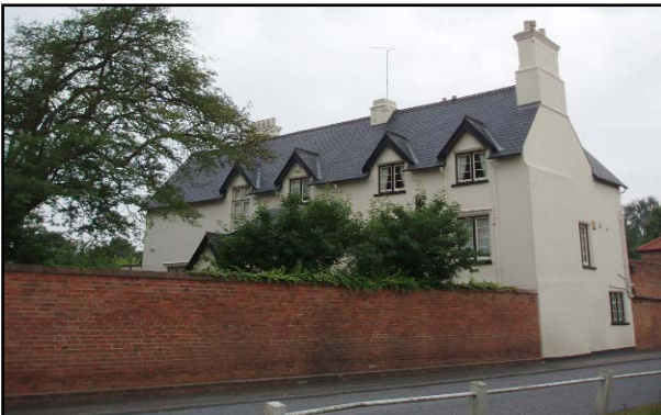
Brick boundary wall on Bleasby Road showing half round copings
