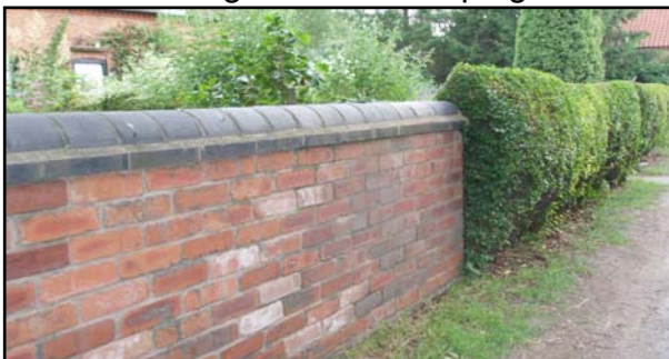
Brick boundary wall on Bleasby Road showing half round copings
