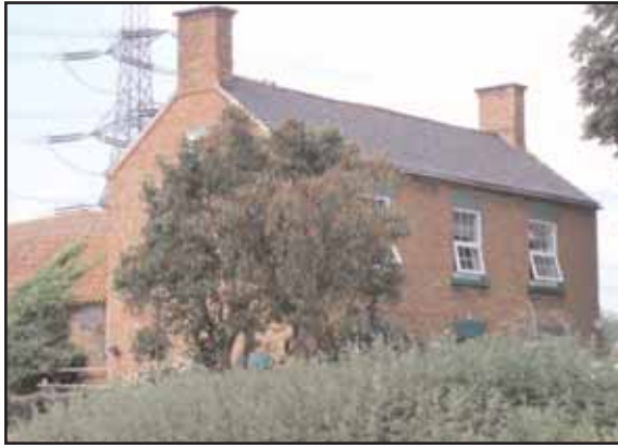
Holly Farm with replacement windows
