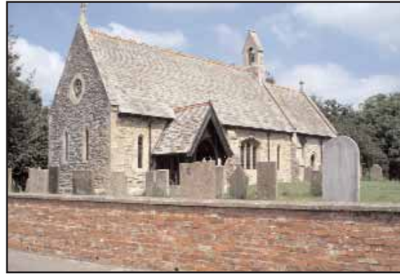
The unusual roof covering on the Parish Church
