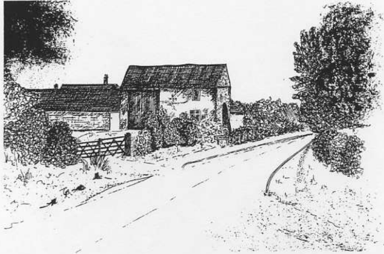
Threshing Barn, Tuxford Road, a good example of an agricultural building which is prominent on one of the approaches into the village.
