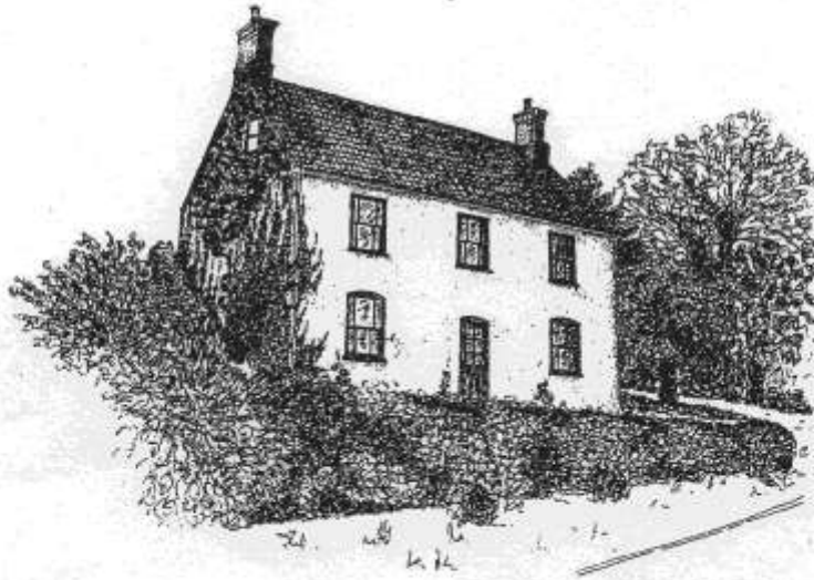
Hollies Farm, Main Street showing the symmetrically arranged windows, gable chimney stacks and pantile roof.
