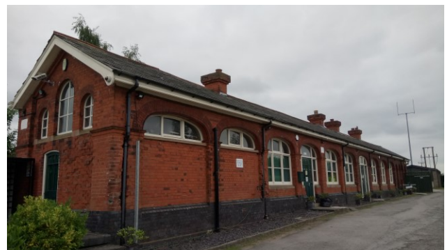
MAIN STATION BUILDING.
