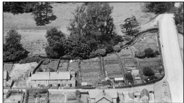
FORMER ALLOTMENTS ON MILL LANE.
