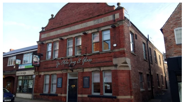
POSITIVE FEATURES. From top: former Methodist Chapel; remnants of the village lock-up; the Old Library; and the former Jug and Glass.
