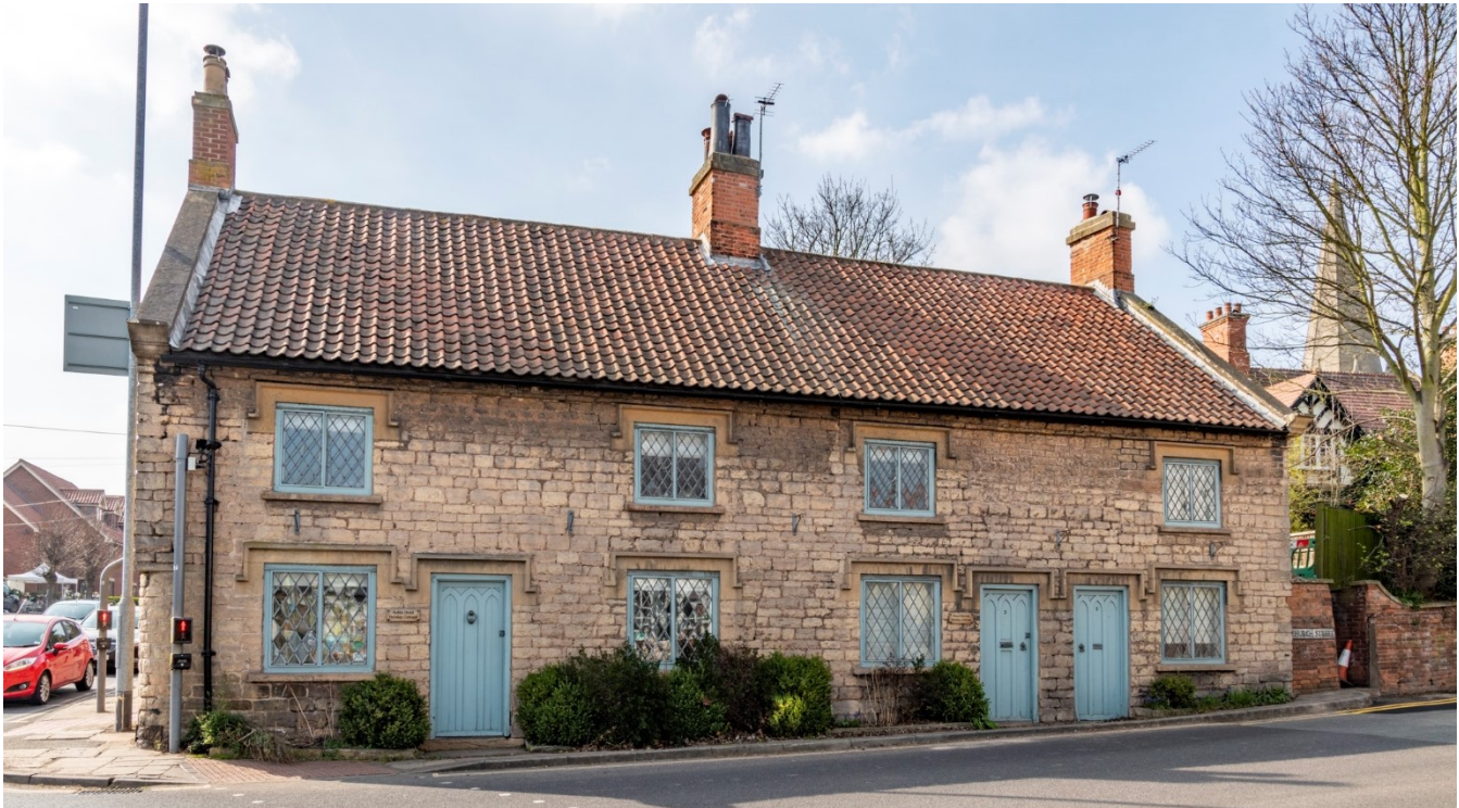
1, 3 AND 5 CHURCH STREET. A row of early 19 th century cottages comprising coursed squared rubble and brick with a clay pantile roof, coped gables with kneelers and latted iron casement windows with distinctive plain hood moulds. The doors have lancet panels and hood moulds.
