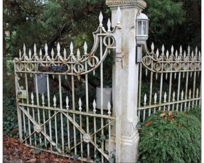
Listed Gate: This area is home to several listed structures, including this gate at the front Kingswood.
