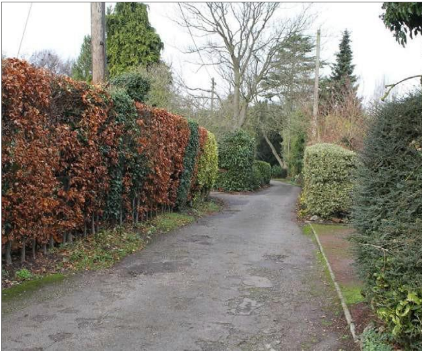
Shared surface: In places with very low vehicle movements (less than 100 per day) it may be appropriate to create a shared surface lane like this one.
