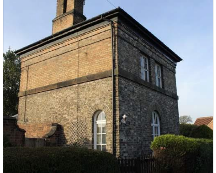
Significant markers: Where variation does occur, it has a logic due to the significance of the structures.
