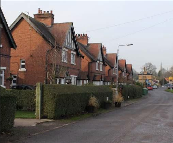
Defining the street: Ordered, regular buildings and a green boundary form a strong edge to the street.
