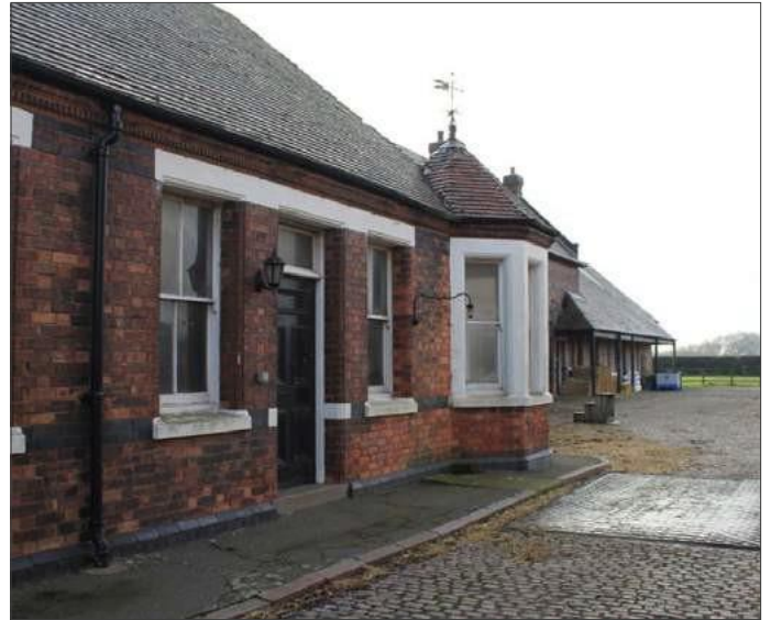
Fine-grained detailing: Simple buildings from the Victorian era still have a rich, fine-grained detailing that add quality when viewed up close.
