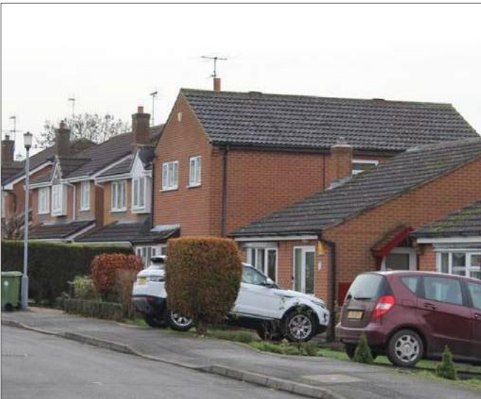
Open plots: The lack of boundaries between plots and streets causes parked cars to dominate the street scene.
