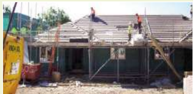
Construction of the new slate tiled roofs on the bungalows.
