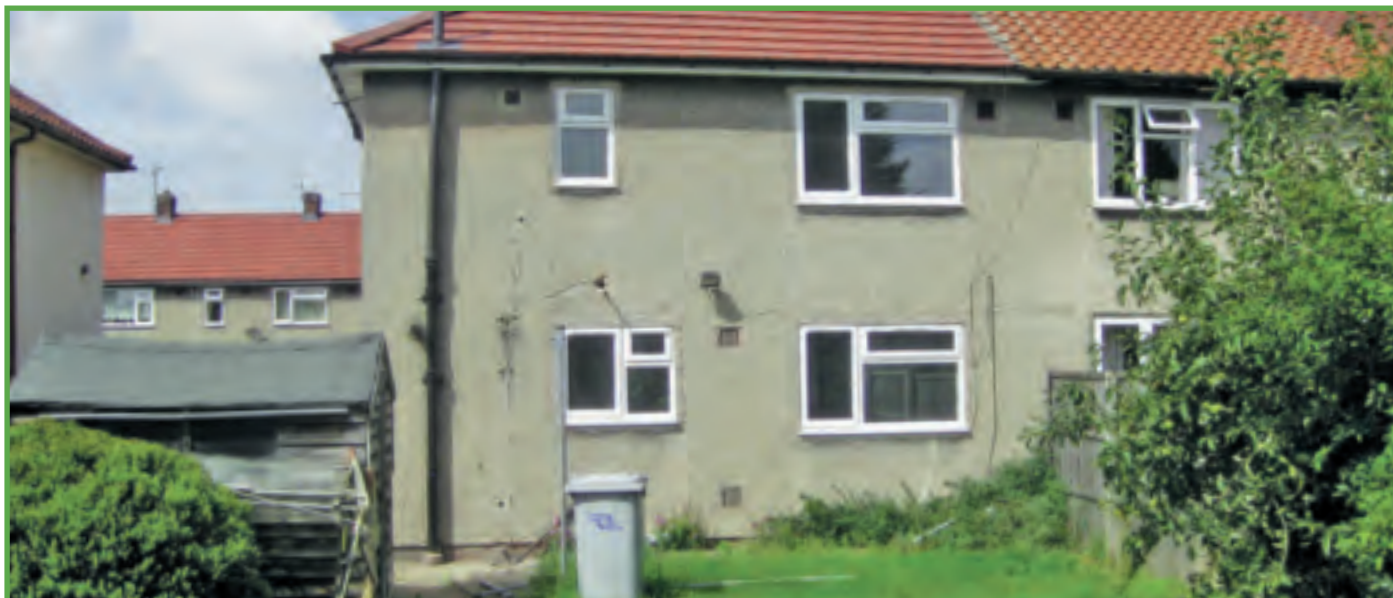
A typical 'no fines' home on Hawtonville
